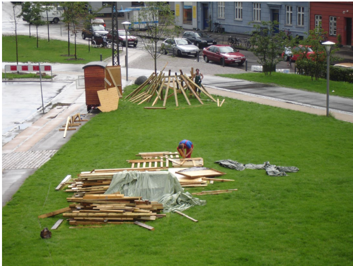
Fig. 1: Beginning the process of construction.
